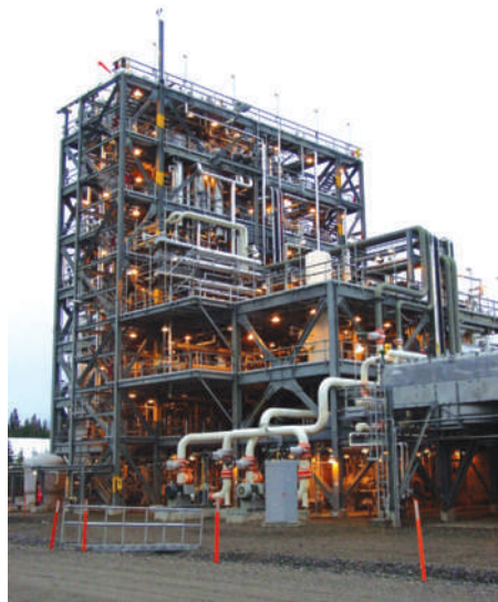
Figure 1 | A Fischer-Tropsch plant. The conversion of coal into liquid fuel via the Fischer-Tropsch process could prove to be one of the most environmentally friendly technologies of the future.
