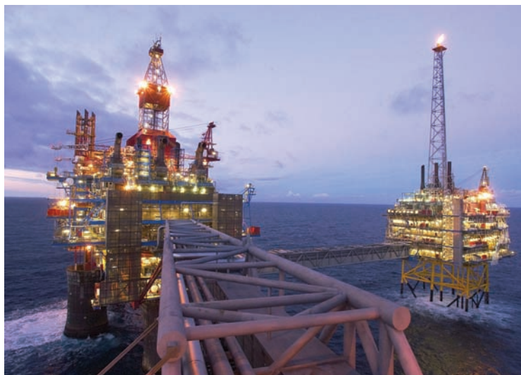
Fig. 1. Since 1996, StatoilHydro has been separating 1 million metric tons of CO 2 per year from a natural gas platform in the Sleipner Field in the North Sea and injecting it into a sandstone reservoir. Seismic monitoring has shown that the CO 2 is safely contained beneath a thick sequence of impermeable shales. [Photo: Dag Myrestrand/StatoilHydro]
