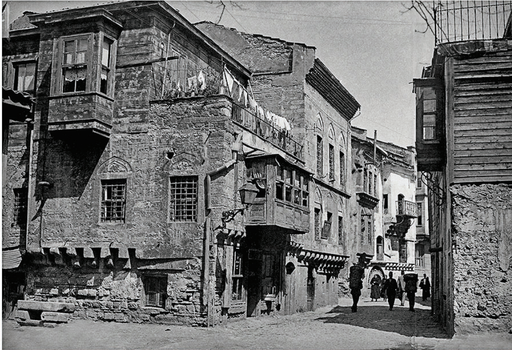
FIGURE 8.4 The Main Street of Phanar (Fener), “Anthology of Phanariot Architecture”, photograph by Achilles Samandji, c.1920
