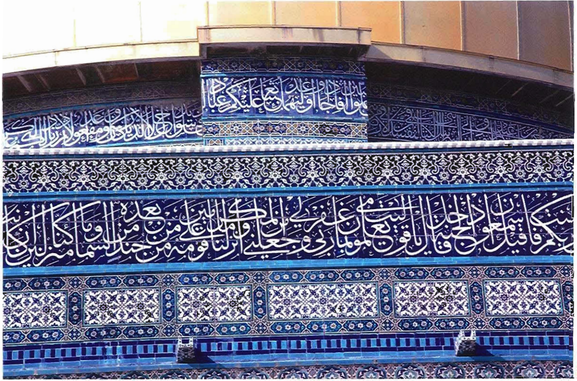
Fig. 18. Dome of the Rock, external tile revetments with inscription bands on the drum and octagon. (Photo: Charles & Josette Lanars/Corbis)
