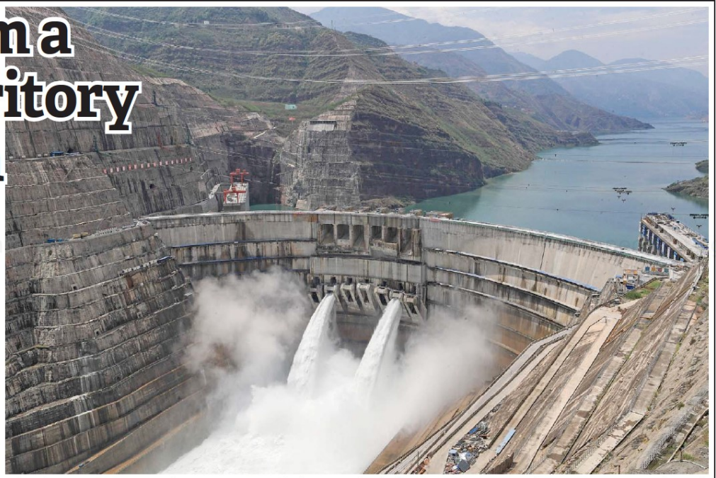
This aerial photo shows the 289m Baihetan Hydropower Station in Zhaotong, in China's south-western Yunnan Province. Hydropower plays a major role in Yunnan's transformation – as at end of 2022, the province possessed an installed hydropower capacity of 81 GW, second only to Sichuan. — AFP photo
