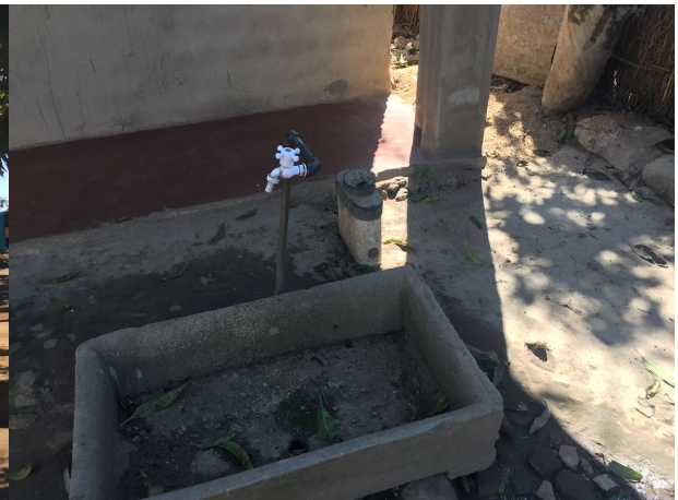
(b) Domestic Low Water Connection
