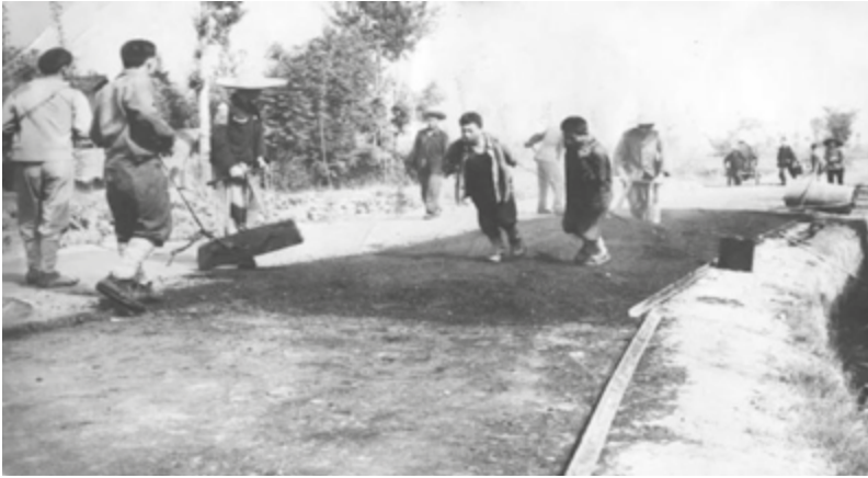
Figure 3. Building a road for a Third Front factory. Source: “‘三线文化’ 三线建设部分老照片选登” [“Third Front Culture”: Select Published Old Photos of Third Front Construction]. 每日头条 [Meiri Toutiao], 20 August 2017, available online at: kknews.cc/zh-cn/news/a8jbqa6.html .
