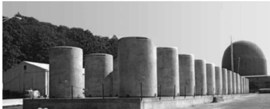
Figure 15. Dry cask storage of older spent fuel at a U.S. nuclear power plant. A 1000-MWe light-water reactor typically annually discharges spent fuel that originally contained about 20 tons of uranium. Each cask typically holds about ten tons and costs $100,000-200,000 per ton of contained spent fuel. Reprocessing a ton of spent fuel would cost $1-3 million [Connecticut Yankee, 2008].
