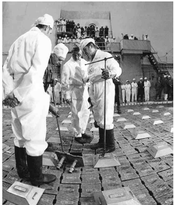
Fig. 7 Top of one of the shut-down Krasnoyarsk-26 reactors. Each square covers one channel. The raised covers indicate the locations of control rods. The two pipe tops show the diameter of the fuel channels. 7
