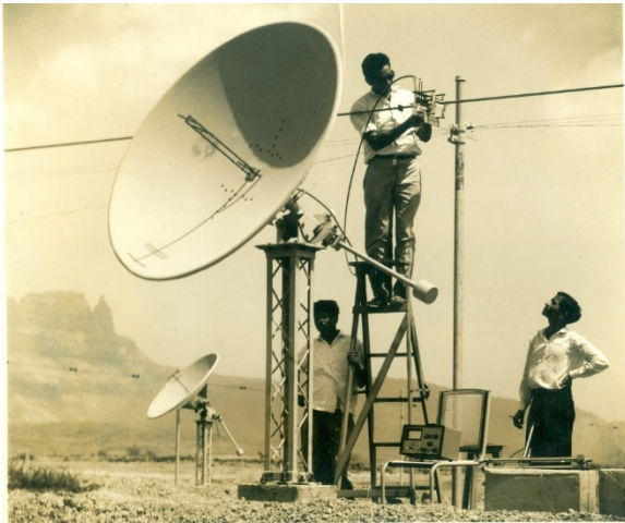
WO Figure 4. RT Kapahi adjusting the transmission line.
