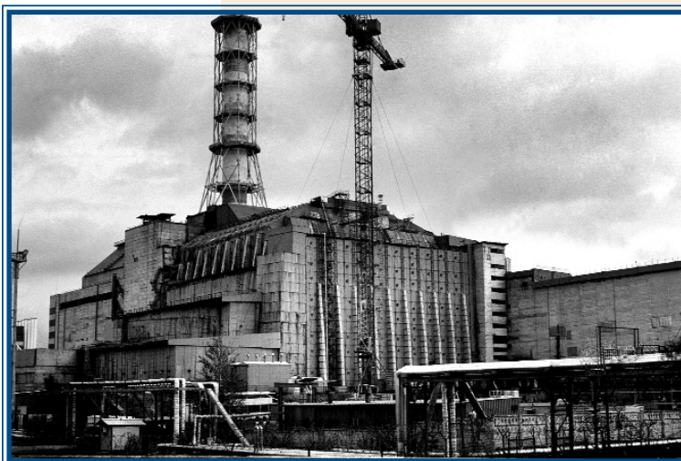
Reactor #4 of the Chernobyl Nuclear Power Plant under the sarcophagus built after the disaster. (Source: Julien Behal/Chernobyl Children's Project)
